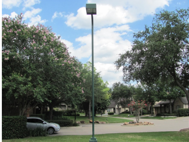
Light pole and fixture at sport court
