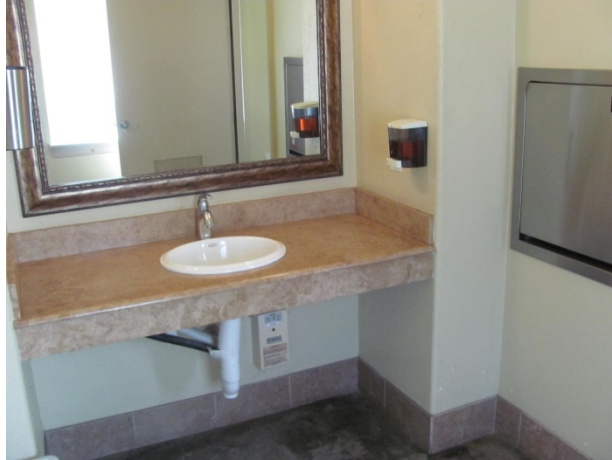
Rest room finishes
