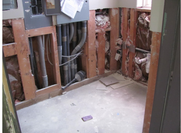
Interior of main guard house currently under renovation
