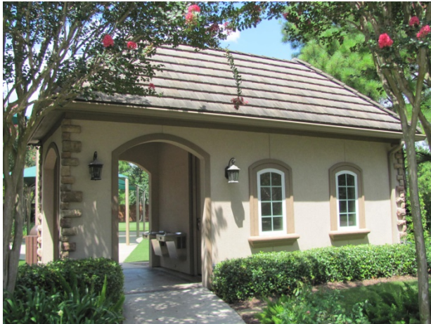
Rest room building at playground
