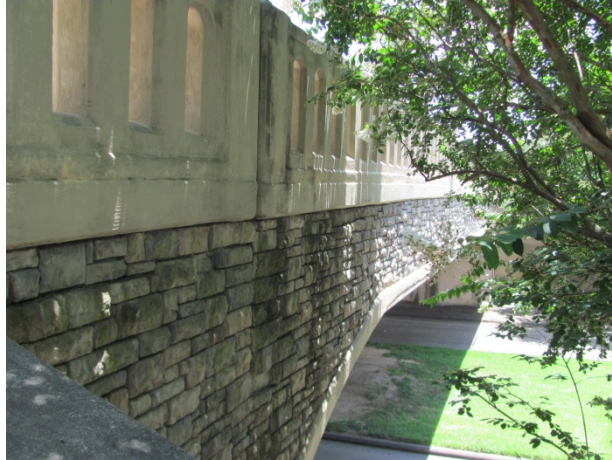
Bridge at Royal Oaks Club Drive over Richmond Avenue
