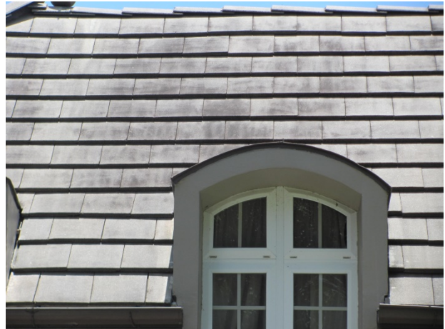
Tiles at main guard house
