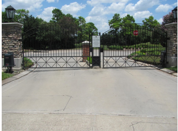
Entry and exit gates at Empress Oaks
