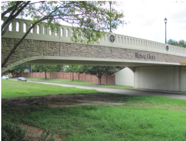
Bridge at Bonnebridge Way Boulevard over Westpark Drive
