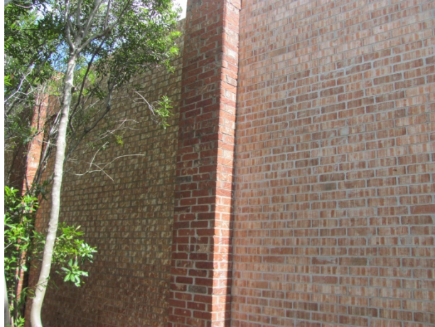
Taller wall at south perimeter
